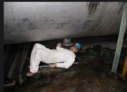
Technicians provide Velometer testing and welding inspection for various projects.
