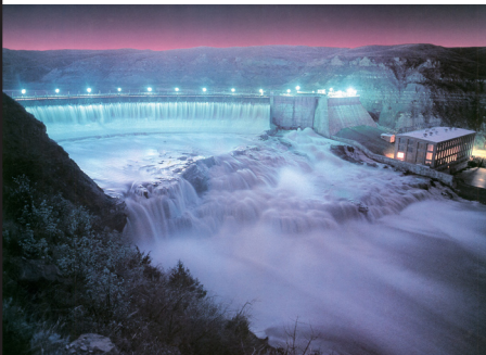
SCADA Plant Control System at Ryan Dam, Montana
