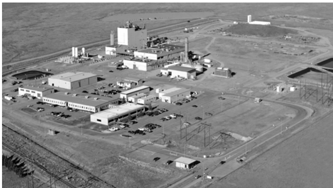
Figure 1. Mike Mansfield Advanced Technology Center.
