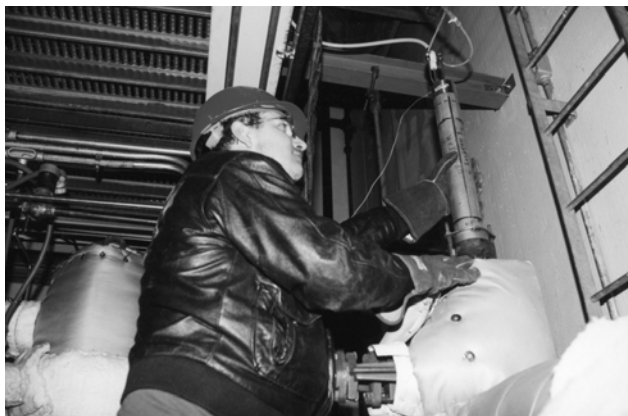
Figure 3. MSE personnel performing stack sampling.
